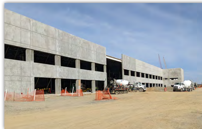
Image of Toyota Megasite under construction
